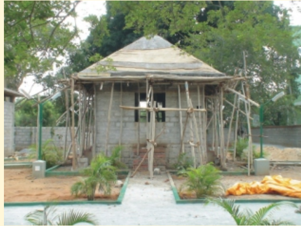
The Temple of Light under construction.
