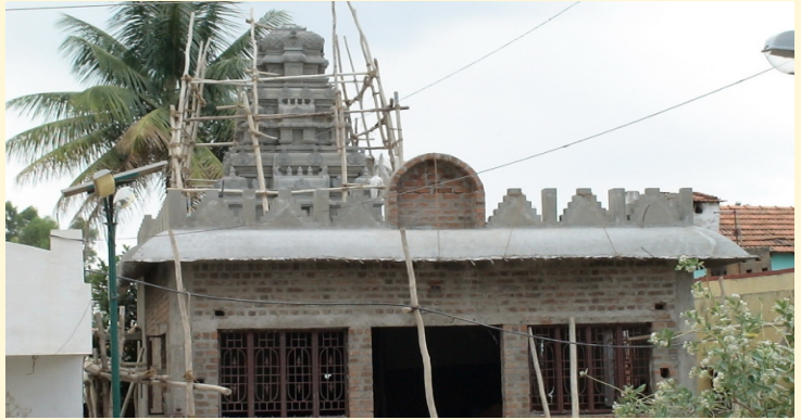
Yellamma Temple under construction at NG Gollahalli.
