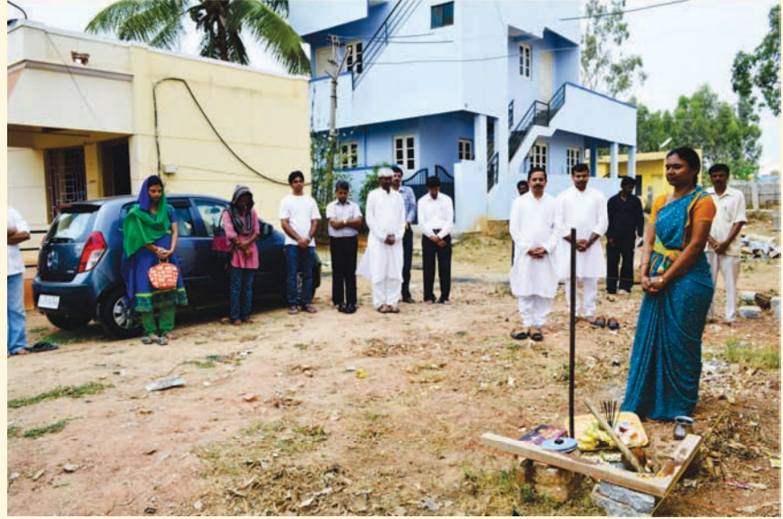
Construction work of the new Light Channels office began on 14th April.
