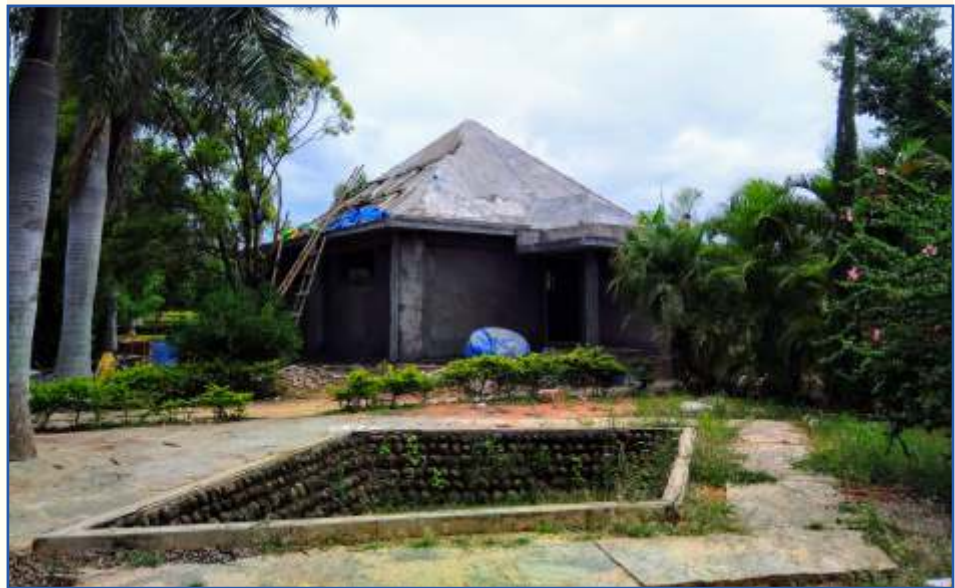
Renovation of Gururji's Samadhi Hall in progress.
