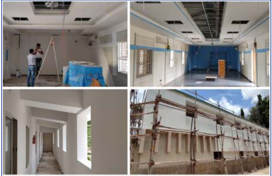
Renovation work of the Meditation hall at Taponagara in progress.
